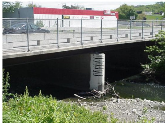
BRIDGE AND CREEK VIEW
